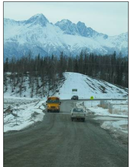
France Road, looking south
